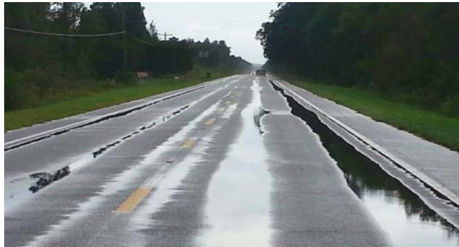
Figure 1.2: Developed ruts in HMA Course.
